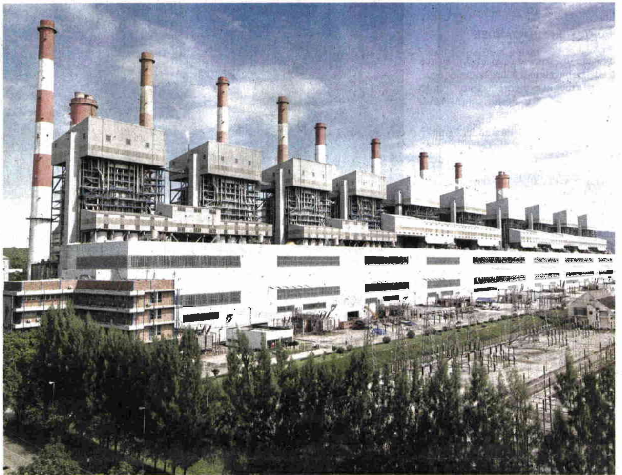
The Mae Moh power plant in Lampang province has been operating since 1975. Upgrades will improve capacity by 300MW per unit.
