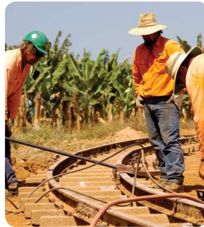
Off season maintenance of the cane rail network, Bundaberg
